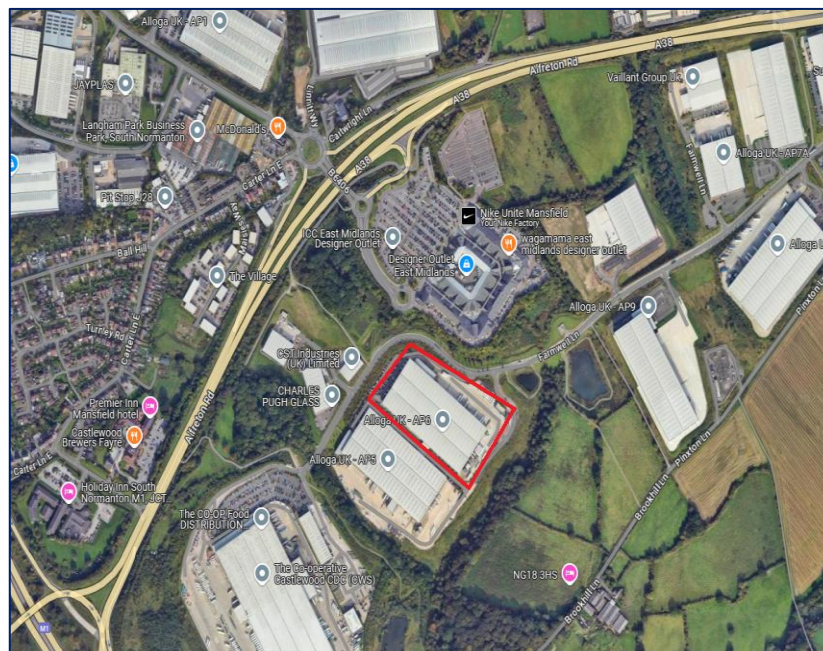
Plot C1 Castlewood Business Park, South Normanton
